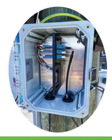
**Small Cell Fiber Jumpers** are intended to interface with Remote Radio Unit (RRU) manufacturers such as Ericsson, Nokia, and Samsung. These versatile jumpers can be used for various applications, such as 5G networks, Distibuted Antenna System (DAS) systems, and Fiber-To-The-Antenna (FTTA).
